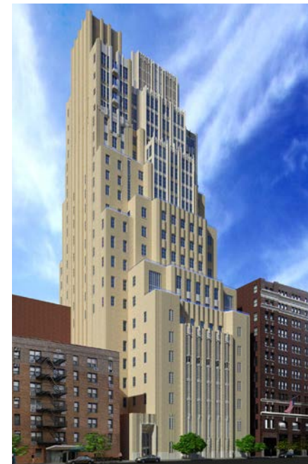
WALKER TOWER, NEW YORK CITY
