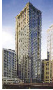
Leo Burnett Building, Chicago, SOF IV
