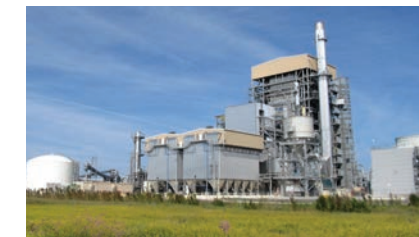
▲ Gainesville Renewable Energy Center, Gainesville, Florida : A 100-megawatt, wood-fired power plant—one of the largest biomass power plants in the U.S.
