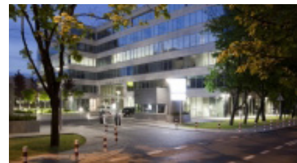
▲ Lopuszanska Business Park, Warsaw : BREEAM Very Good certification.
