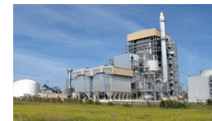
▲ Gainesville Renewable Energy Center, Gainesville, Florida : A 100-megawatt, wood-fired power plant—one of the largest biomass power plants in the U.S.
