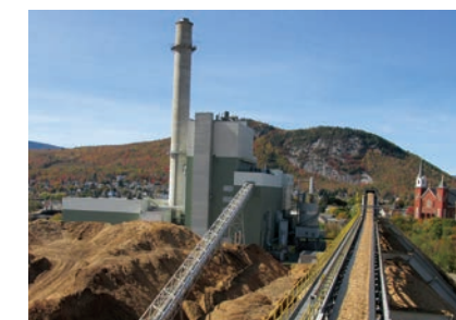
▲ Berlin Station, Berlin, New Hampshire : A 75-megawatt, wood-fired power plant—one of the largest biomass power plants in the Northeast.
