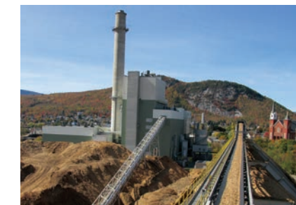
▲ Berlin Station, Berlin, New Hampshire : A 75-megawatt, wood-fired power plant—one of the largest biomass power plants in the Northeast.
