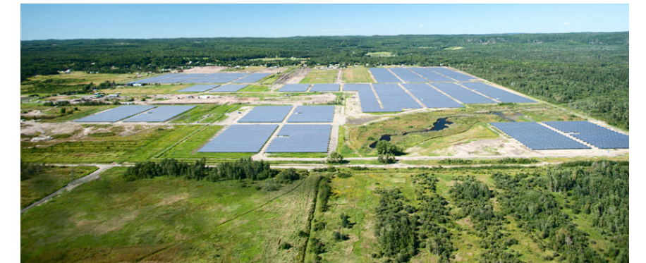
▲ Starwood Solar Sault Ste. Marie, Ontario, Canada : A three-phase, 69-megawatt DC solar photovoltaic project—one of the largest solar power plants in Canada.
